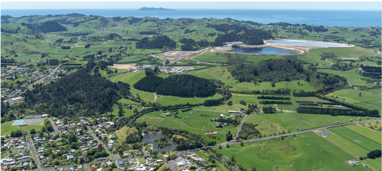
Aerial view of OceanaGold Waihi Operation tailings storage facility.
